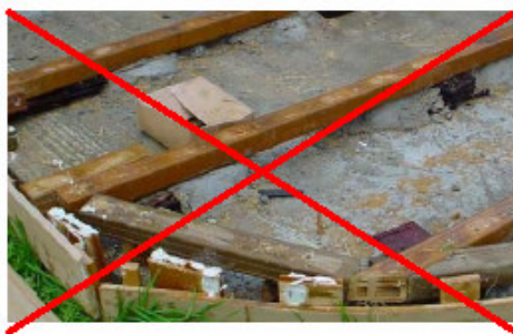
Leave 10 mm space between ends when butting the bearers
