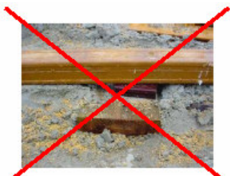
Do not seal bearers in concrete
