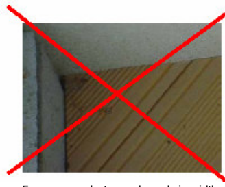
Leave 5 mm space between boards in width and 15 mm between the board end and the wall.
